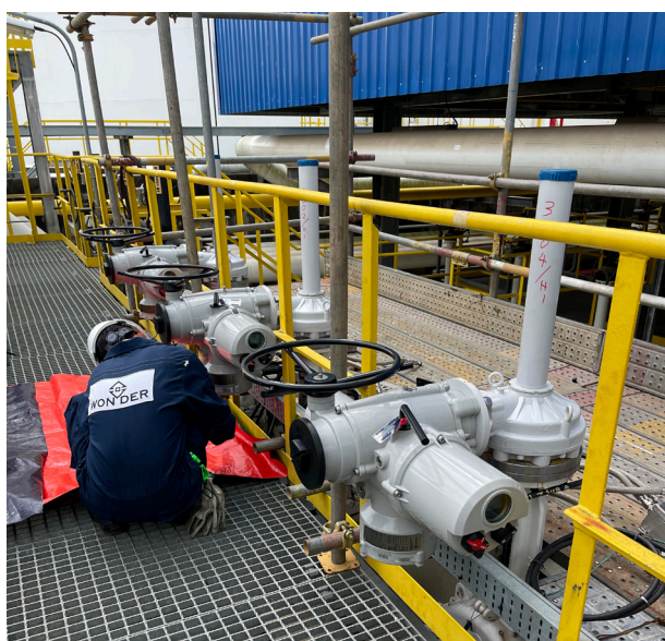
Figure 1. Field commissioning of Wonder MOV actuators.
