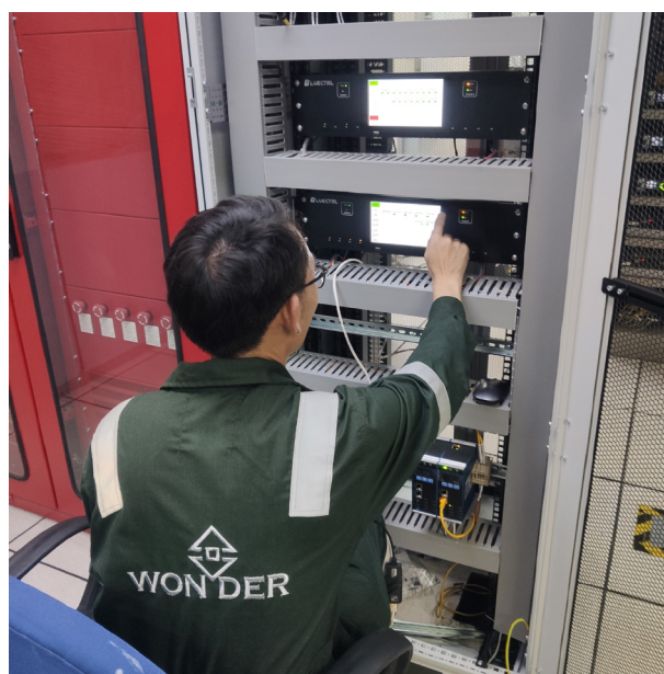
Figure 2. Field configuration for master station using Modbus RTU (RS-485).
